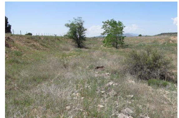
Photo 9. Embankment and concrete piles in Arroyo de las Calabasas
